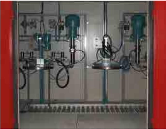
Installation of 2 paint supplies in container
