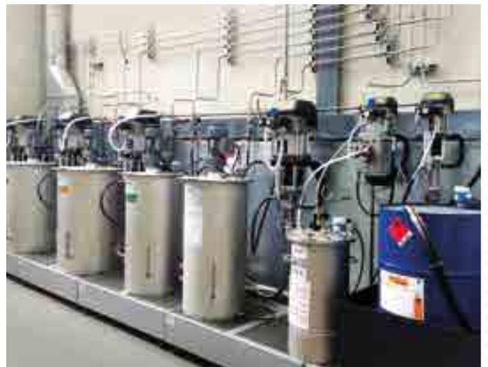
... and after: Central paint supply with WALTHER PILOT paint mixing tanks type FMB: Only one hardener (MDG 45) required for all materials.
