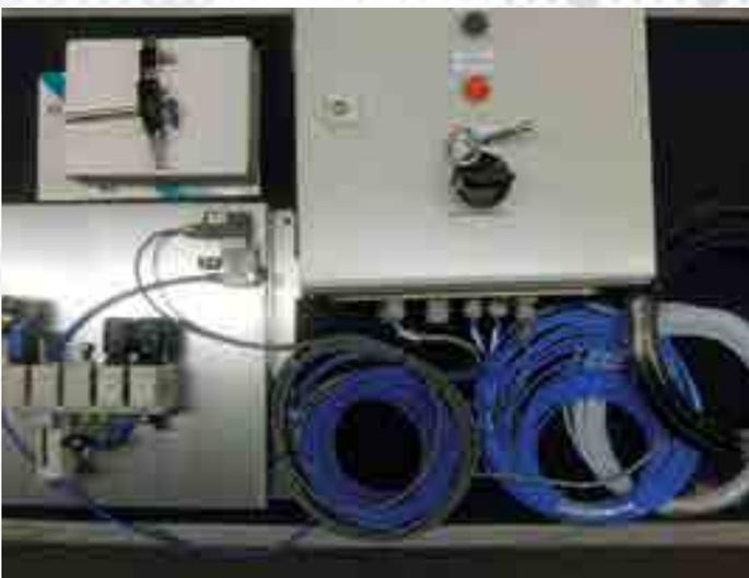
Marking gun control on mounting plate
